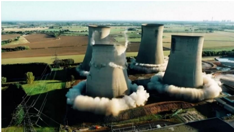
Figure 7: Demolition of Eggborough coal-fired power station (source: CNN)
