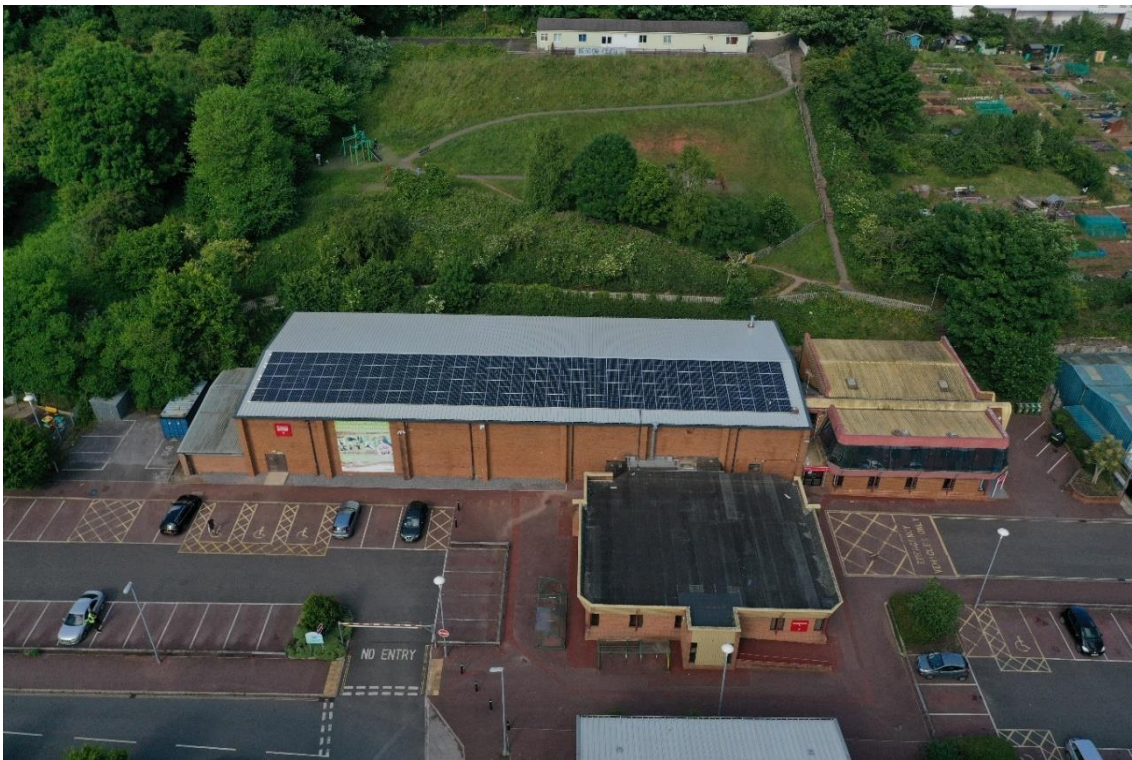
Figure 23: Aerial view of Broadmeadow Sports Centre
