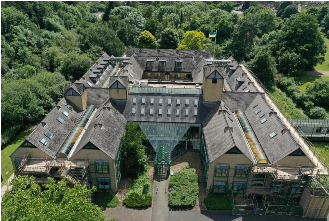
Figure 21: Aerial view of Forde House
