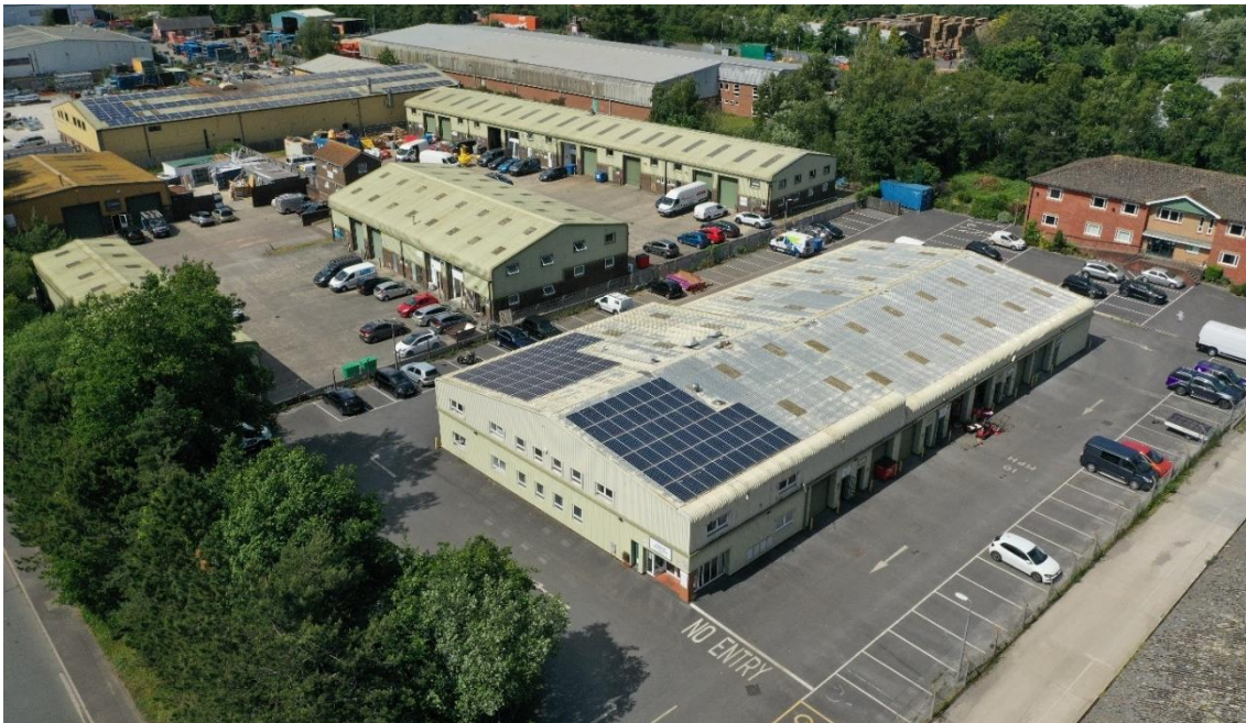
Figure 30: Aerial view of the Teignbridge Business Centre
