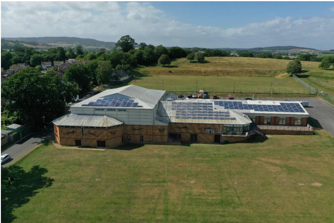
Figure 22: Aerial view of Dawlish Leisure Centre
