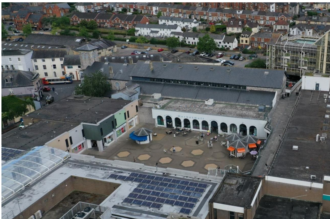
Figure 25: Aerial view of Market Hall
