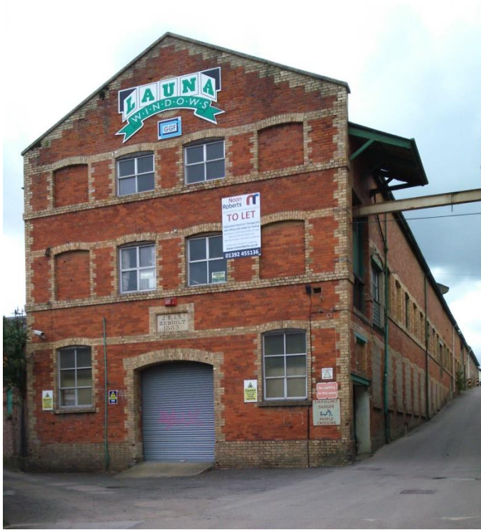
The Fleece Shed, one time “Launa Windows” building
