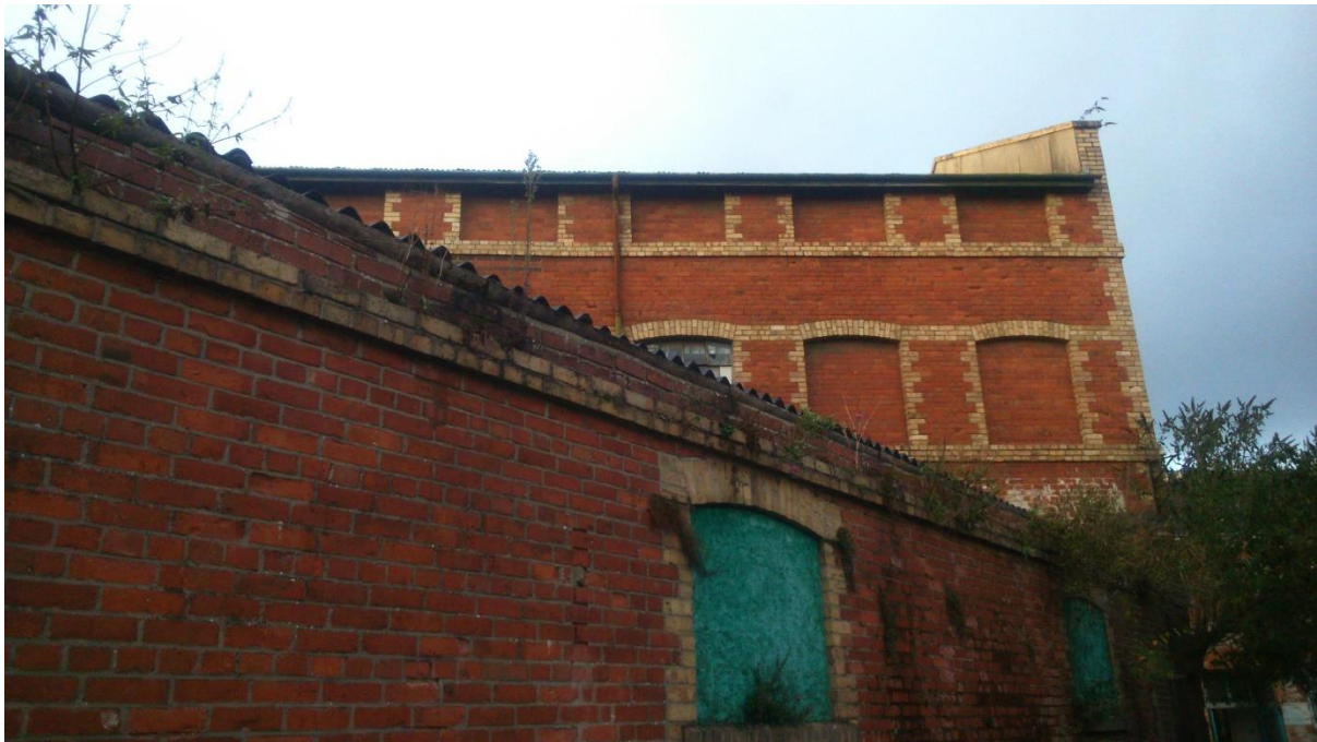
Rear/South wall at eastern end
