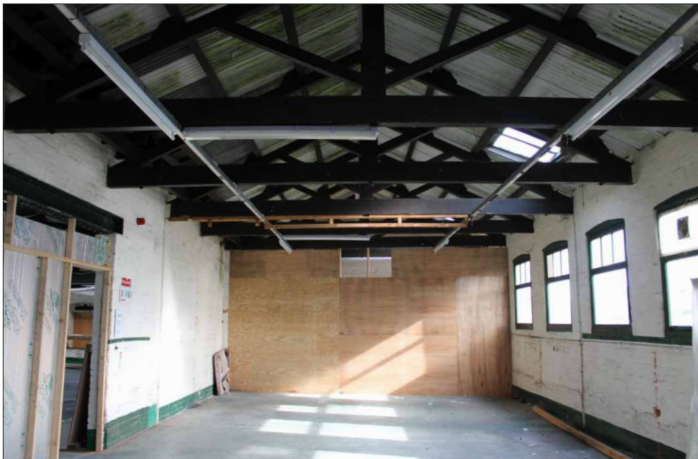
Plate 16: Internal view of structure 8, looking northeast
