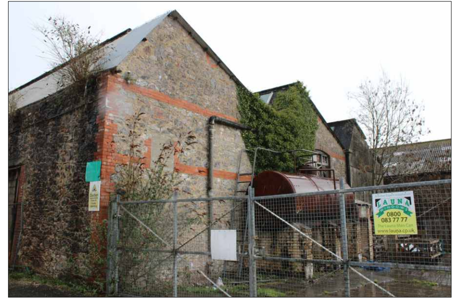
Plate 21: General view of the southern buildings, looking northeast
