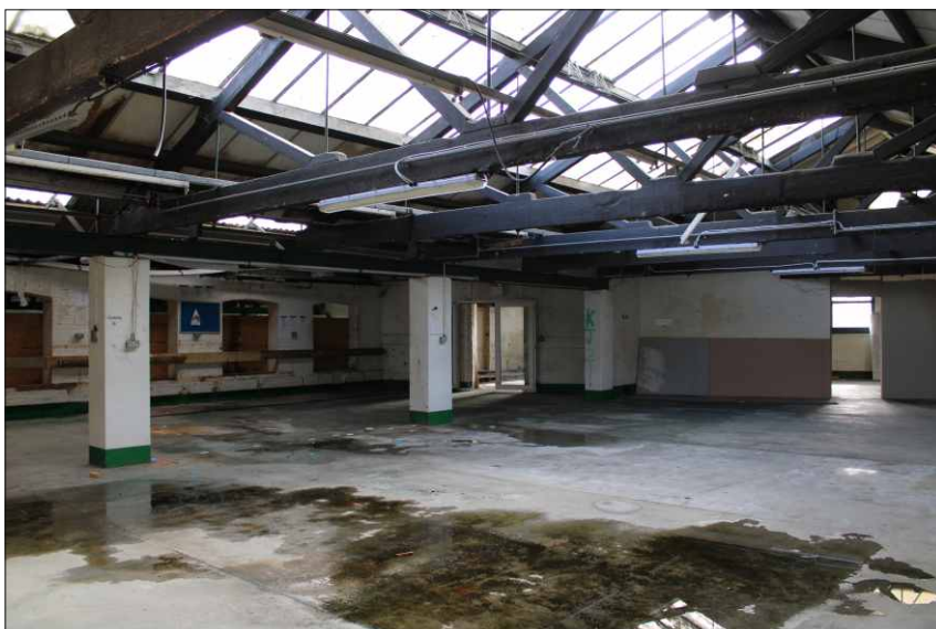
Plate 14: Internal view of structure 7, view towards structures 8 and 9, looking southeast
