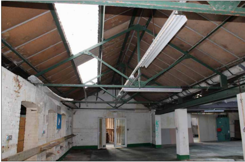
Plate 17: Internal view of structure 9, looking southeast
