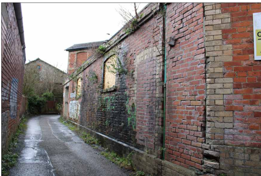
Plate 19: East elevation of structure 11, looking south
