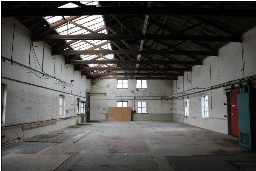
Plate 3: Internal view of structure 1, looking northeast
