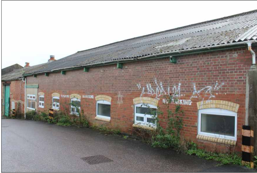
Plate 6: North elevation of structure 3, looking southeast
