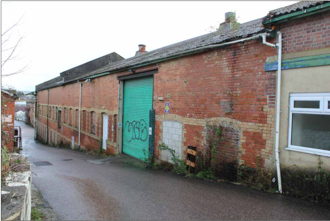
Plate 4: North elevation of structure 2, looking east
