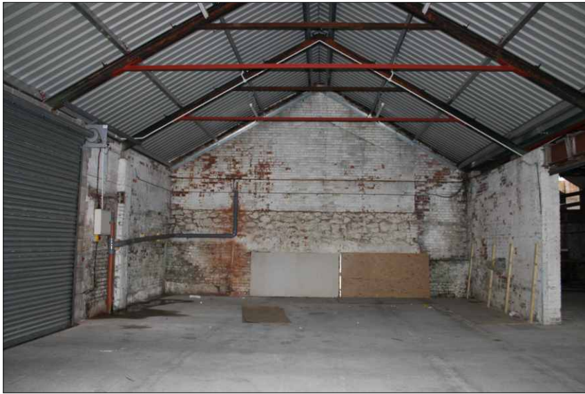
Plate 12: Internal view of structure 5, showing earlier roof line, looking north
