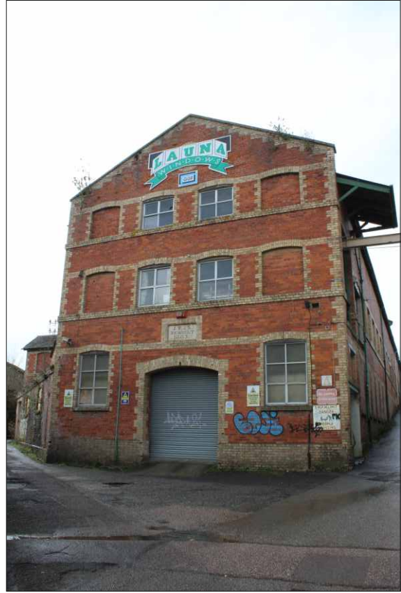
Plate 2: East elevation of structure 1, looking southwest
