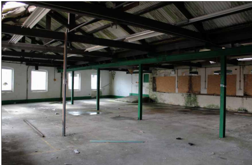
Plate 18: Internal view of structure 10, looking south
