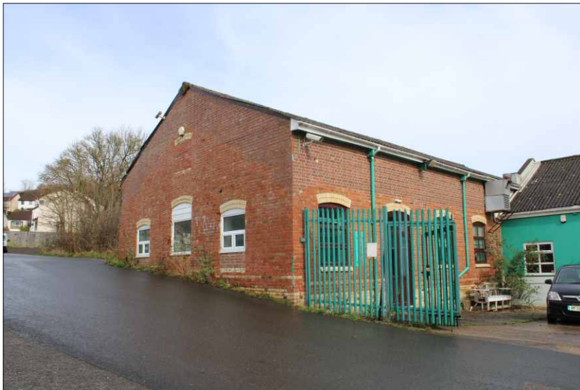
Plate 7: South and west elevations of structure 3, looking north
