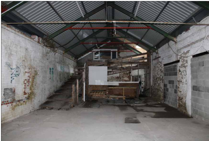
Plate 13: Internal view of structure 6, looking north
