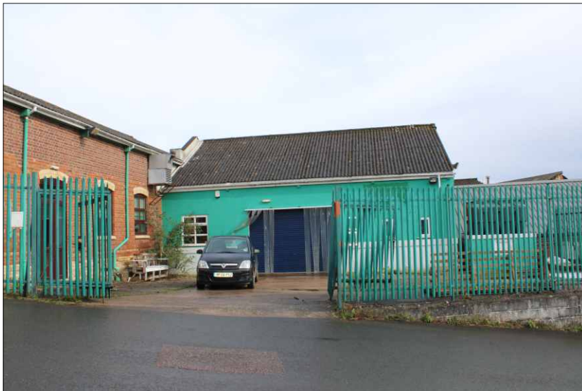
Plate 10: West elevation of structure 4, looking northeast
