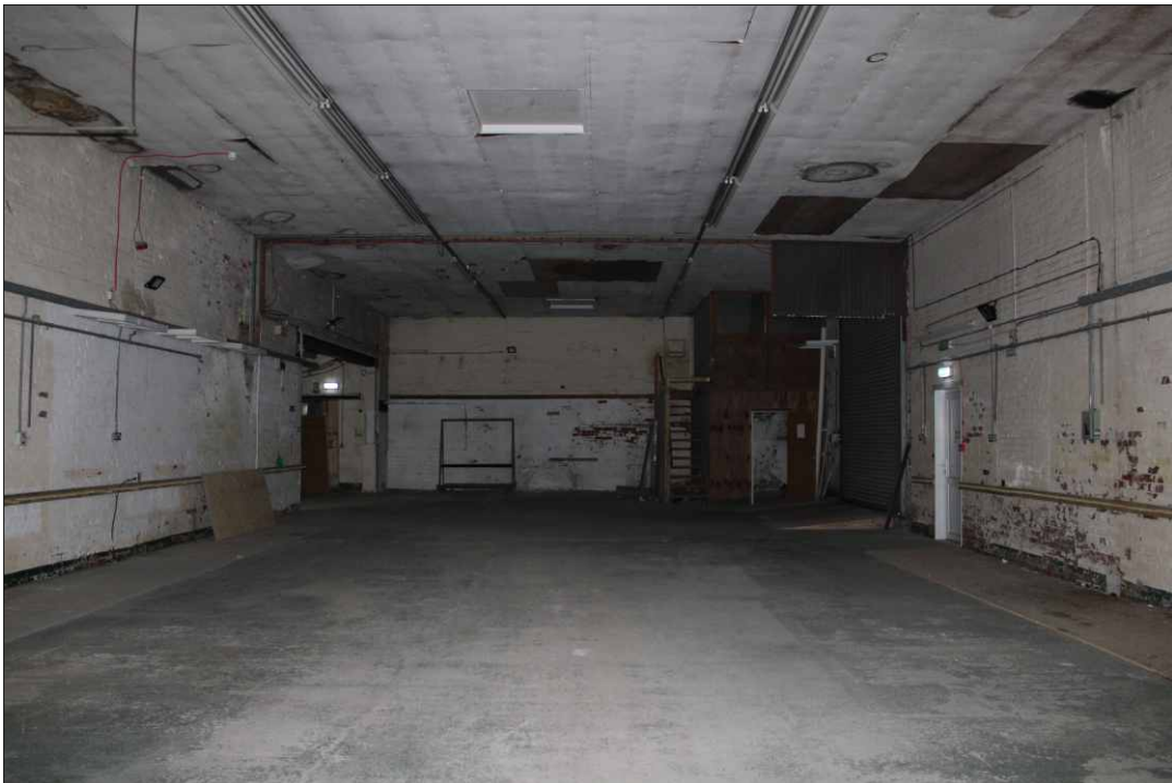
Plate 5: Internal view of structure 2, looking southwest
