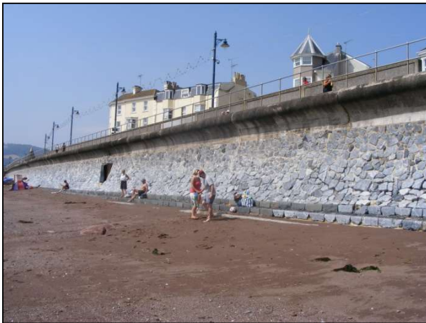
Figure 2.13 Rock-faced, concrete seawall constructed in the mid 1970's.
