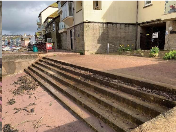
3934 Concrete quay and steps fronting Morgans Quay properties with low levels doors and openings through properties.
