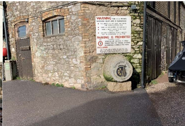
4142 Flood defence alignment appears to run through the Garstone Garden Ornaments property. Not inspected.
