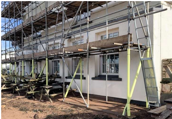
392734 Property wall of the New Quay Public House in good condition, windows do not appear to be floodproof.
