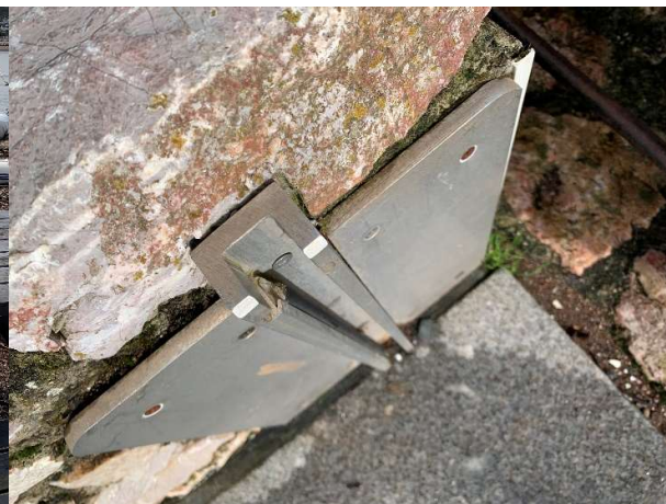
524451 End channels secure and in very good condition.
