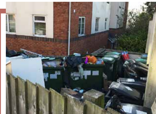
Bin stores need to be properly designed to avoid creating an unsightly and unpleasant environment for residents.
